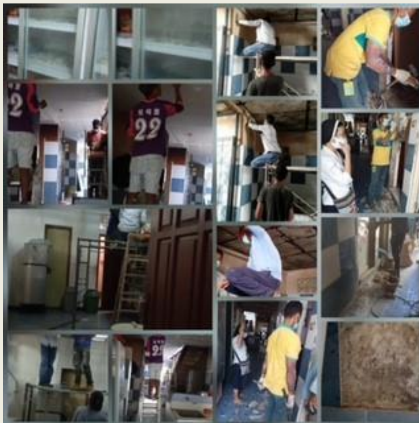
Photo collage of work in progress at the Dominican Orphanage - Bidau
